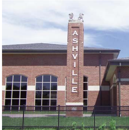
ASHVILLE ELEMENTARY SCHOOL, ASHVILLE, OHIO
