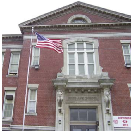
REEB ELEMENTARY SCHOOL, COLUMBUS, OHIO
